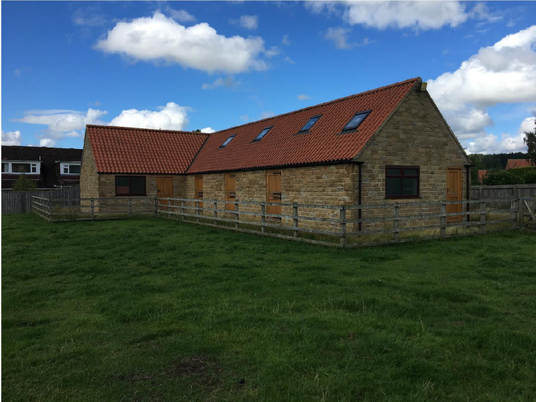
Existing building viewed from the south east and showing the traditional materials and proportions of the structure.
